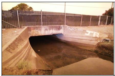
**Inspect ID:** SMNR\_2020\_a\_0005 **Title:** USACE\_CESPN\_SMNR\_2020\_a\_0005\_1.jpg **Rated Item: 5.** Concrete Surfaces **Caption:** Rating: Minimally Acceptable; Remarks: Photo is looking downstream at concrete culvert, Concrete spalling and exposed rebar was observed on the culvert entrance. Action: The Sponsor should initiate the repair as soon as possible to prevent further deterioration.; Station: 19+00
