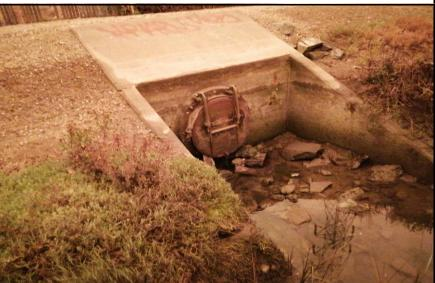
**Inspect ID:** SMNR\_2020\_a\_0004 **Title:** USACE\_CESPN\_SMNR\_2020\_a\_0004\_1.jpg **Rated Item:** 11. Culverts / Discharge Pipes **Caption:** Rating: Acceptable; Remarks: The culvert flap gate was observed to be in good condition; Action: The Sponsor should perform a video inspection for the culverts every 5 years. At this time the video inspection is not overdue; however, this item should be followed up in next inspection; Station: 19+50
