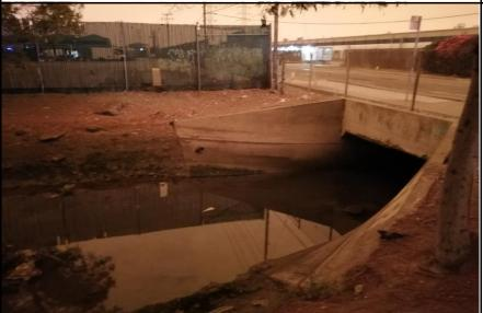
**Inspect ID:** SMNR\_2020\_a\_0005 **Title:** USACE\_CESPN\_SMNR\_2020\_a\_0005\_2.jpg **Rated Item:** 4. Erosion **Caption:** Rating: Minimally Acceptable; Remarks: minor erosion was observed on the bridge wingwalls; Station: 19+00
