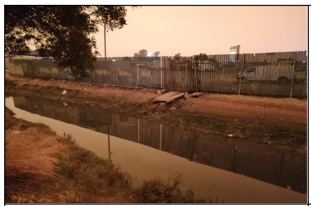
**Inspect ID:** SMNR\_2020\_a\_0006 **Title:** USACE\_CESPN\_SMNR\_2020\_a\_0006\_1.jpg **Rated Item:** 4. Erosion **Caption:** Rating: Minimally Acceptable; Remarks: A broken concrete swale drain that extended from adjacent parking lot to the channel is causing erosion on the channel slope; Action: The Sponsor should repair before the erosion getting larger. Station: 16+00
