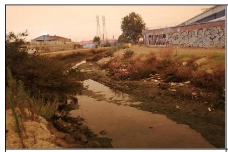
Inspect ID: SMNR\_2020\_a\_0003 Title: USACE\_CESPN\_SMNR\_2020\_a\_0003\_1.jpg Rated Item: 1. Vegetation and Obstructions Caption: Rating: Minimally Acceptable; Remarks: Photo is looking downstream at the channel. A vegetated shoal that spanned approximately 30% of the channel width was observed.; Action: The shoal should be removed if it reduces channel capacity resulting in flood in a high flow event.; Station: 21+00
