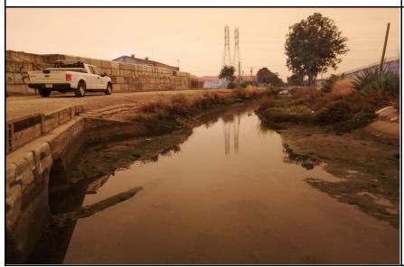
**Inspect ID:** SMNR\_2020\_a\_0002 **Title:** USACE\_CESPN\_SMNR\_2020\_a\_0002\_1.jpg **Rated Item:** 10 Riprap Revetments & Banks **Caption:** Rating: Acceptable; Remarks: Photo shows the upstream of project, looking downstream at the banks, no displaced riprap on side slopes was observed.; Station: 23+00
